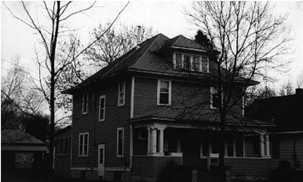
Image 7. Welin House, 430 5 th Ave. SE, BN-SCC-197
