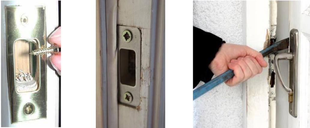
A **heavy duty strike plate** installed in place of a regular strike plate helps strengthen door frames. The heavy duty strike plate uses four to six, three-inch screws and not two, three-fourth inch screws that are typically used in regular strike plates. The longer screws go through the frame into the jamb making it harder for someone to split the frame when kicking the door or applying pressure with an object. A heavy duty strike plate will strengthen the door jamb plus reinforce the lock.
